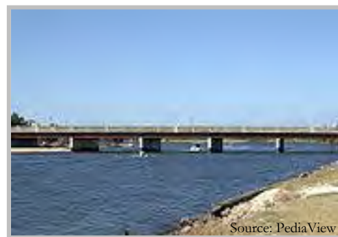
Example of causeway built on piers
