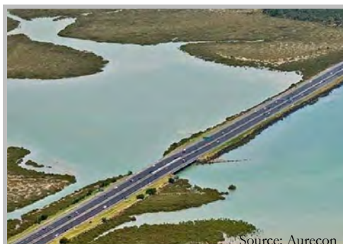
Example of causeway built on a dike
